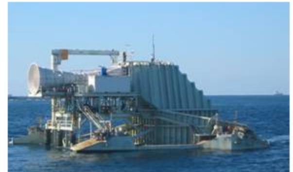
Oscillating Water Column
