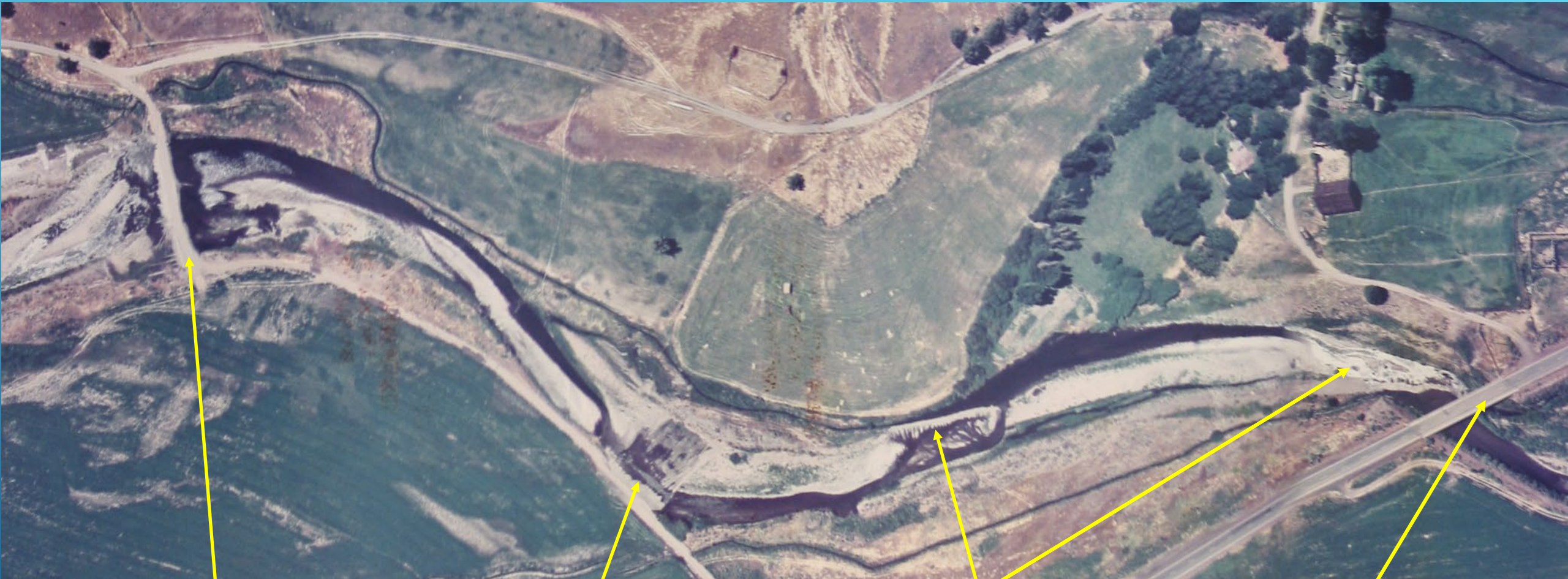
Annual Road Crossing Installation Site
