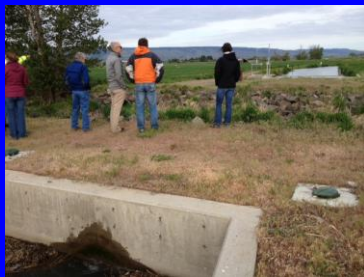
Irrigation canal diverted under creek to avoid fish entrainment in upper Yakima River
