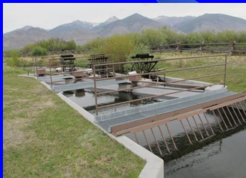
Fish screen in Lemhi River where an estimated 71% of Chinook smolts had been killed by entrainment (Walters et al. 2012)
