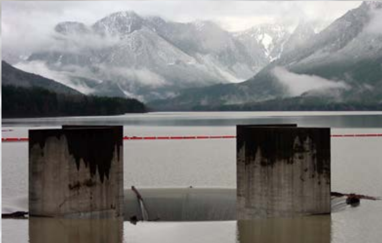
Henry M. Jackson Hydroelectric Project (112 MW)
