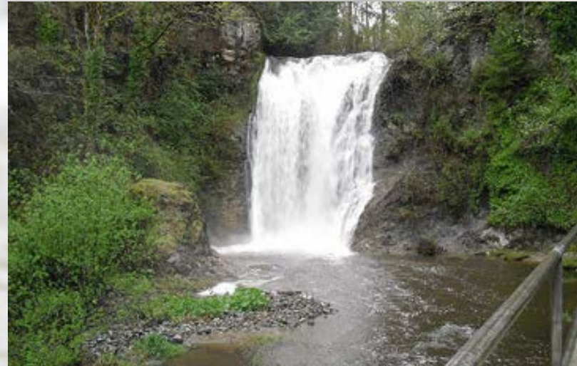
Woods Creek Hydroelectric Project (nameplate capacity of 0.65 MW)
