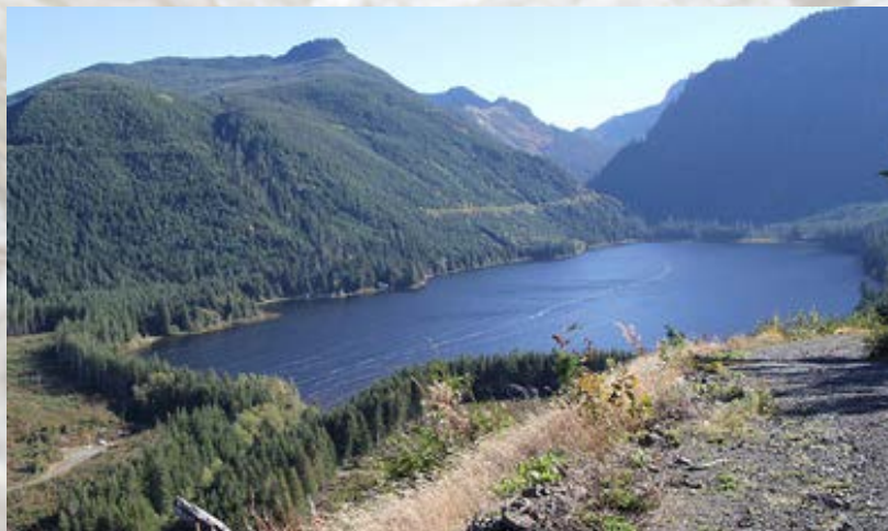
Calligan Creek & Hancock Creek Hydroelectric Projects (6 MW each, under construction)
