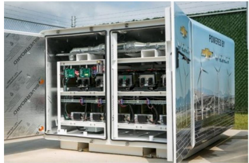
Used Chevrolet Volt batteries are helping keep the lights on at the new General Motors Enterprise Data Center at its Milford Proving Ground in Milford, Michigan. Five Volt batteries work with an adjacent solar array and two wind turbines to help supply power to the data center's administrative offices. (Photo by John F. Martin for General Motors)
