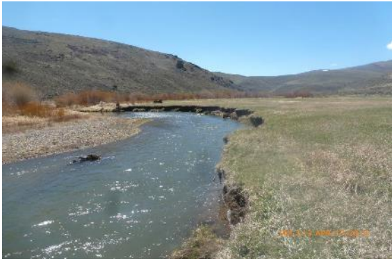
Prior to bank stabilization
