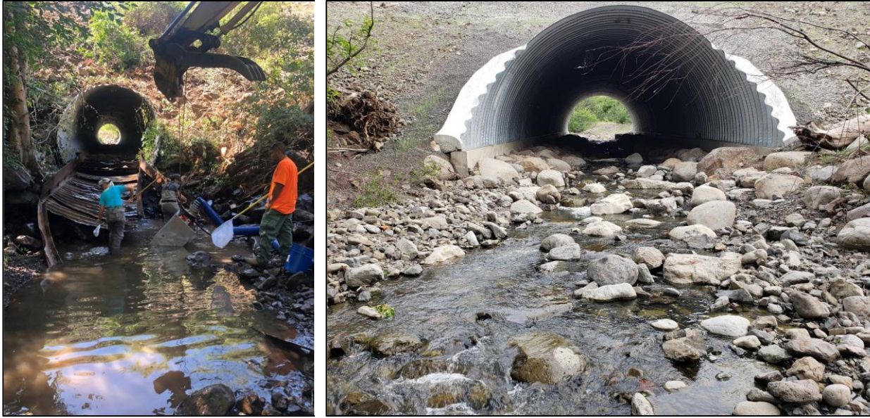
Figure 3.1. Example of culvert replacement to remove a barrier to fish passage, Grande Ronde River/Buford Creek Fish Passage 2019 (Source: FWP project # 2007-393-00 , Nez Perce Tribe).
