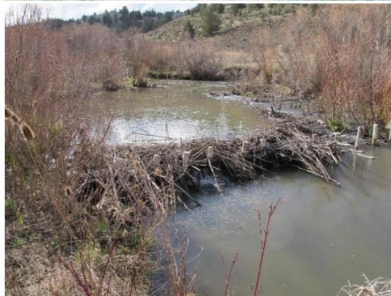
Figure 3.5. Example of beaver dam analogs in Bridge Creek, John Day River subbasin, Oregon. The BDA structures facilitated development of beaver complexes and habitat responses, resulting in increased juvenile steelhead survival and productivity. (FWP project #2003-017-00, NOAA Fisheries, completed) (Sources: aerial photos from PNAMP Bridge Creek IMW Accomplishment Report ; BDA photo from the ISRP).
