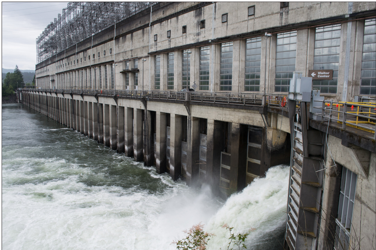
First Powerhouse, Bonneville Dam
