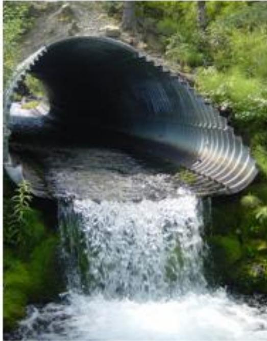
Figure II.10. Poorly designed culverts block upstream fish passage. Photo: Cecil Rich.
