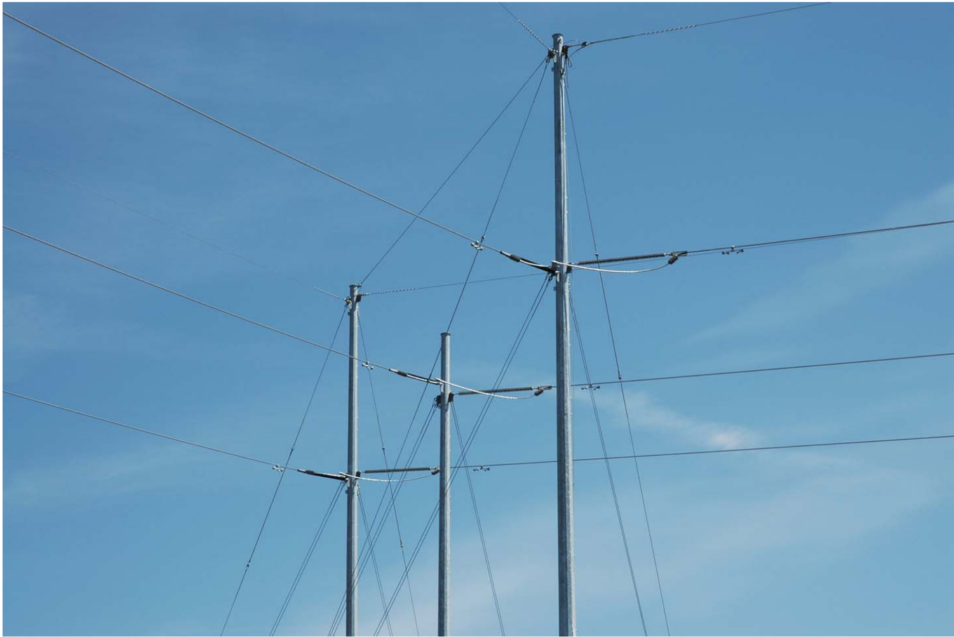
230 kV collector lines will carry Big Horn's output to the Spring Creek switchyard.
