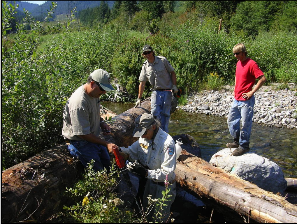
Confederated Tribes of the Warm Springs staff completing log anchoring during first phase of the West Fork Large Wood Addition Project in 2006". Photo by Joe McCanna.
