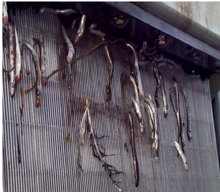
Figure 6. Juvenile lamprey impinged on a mainstem dam VBS.
