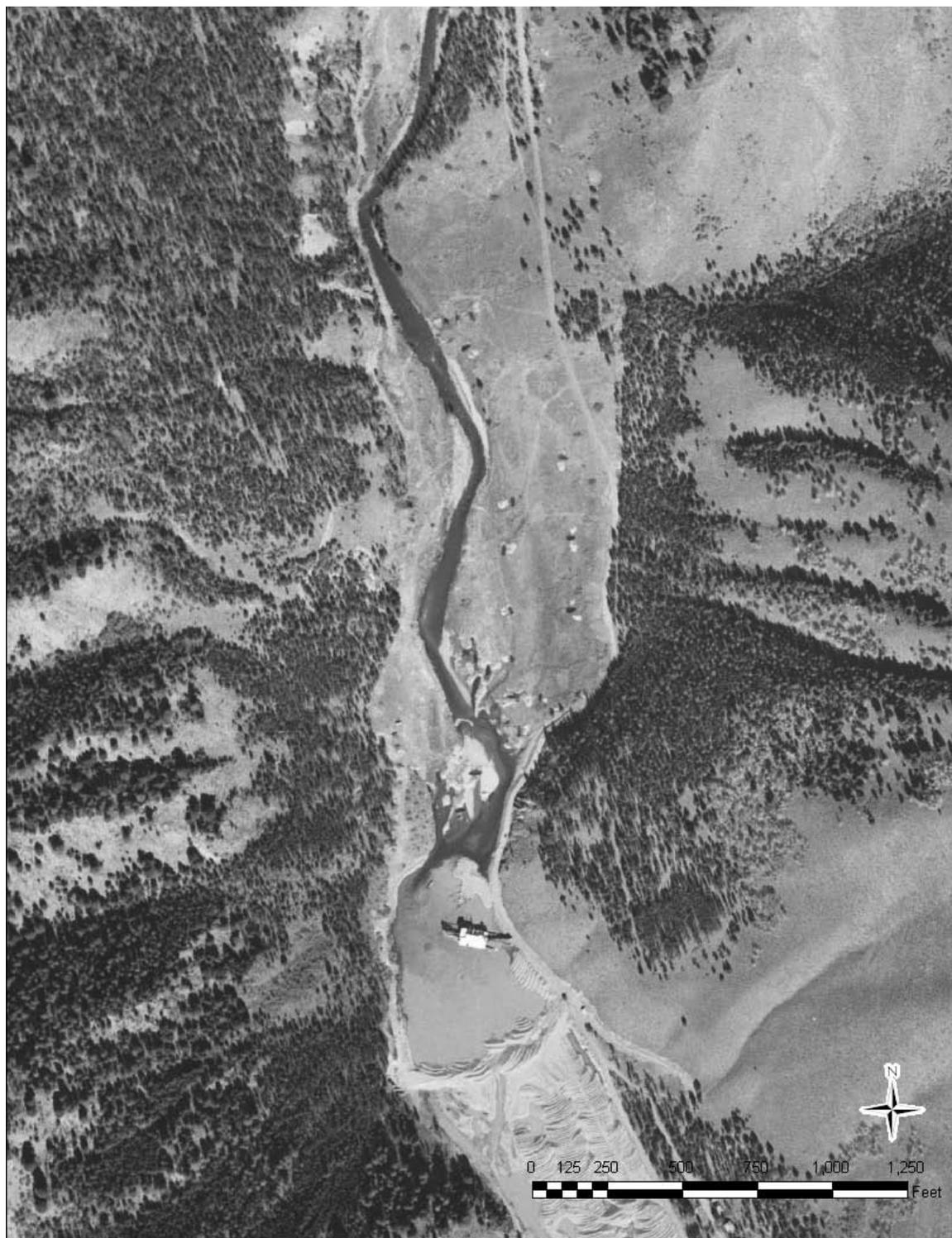
**Figure 36. 1945 aerial photograph of Yankee Fork near Jerrys Creek.** *Note the floating dredge in the lower center of the photograph and the dredge tailings deposited across the valley floor.*
