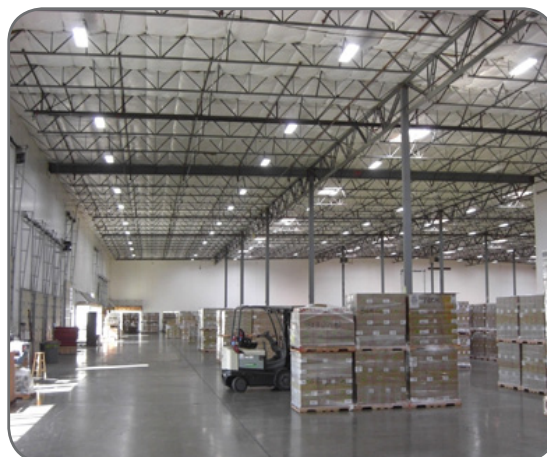
AFTER: T5/HO – 234 watts, 20 foot-candles
