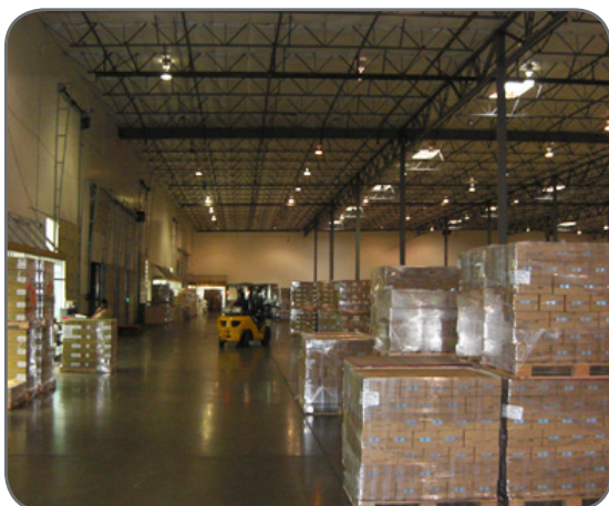
BEFORE: 400 MH – 461 watts, 6 foot-candles
