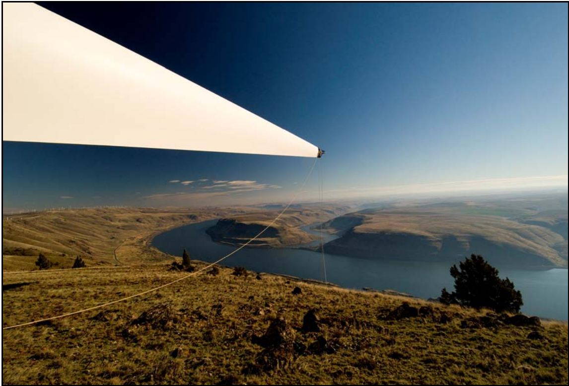
A wind turbine blade is ready to be lifted into place at the Windy Point Wind Farm in the Columbia River Gorge. Photo: C. Bruce Forster
