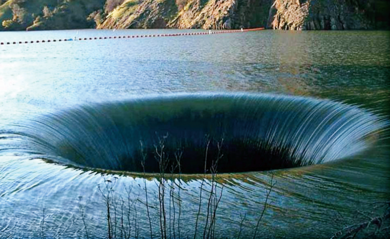
The glory hole spillway at Hungry Horse Dam is the highest in the world. Water cascades over the rim and drops 490 feet.
