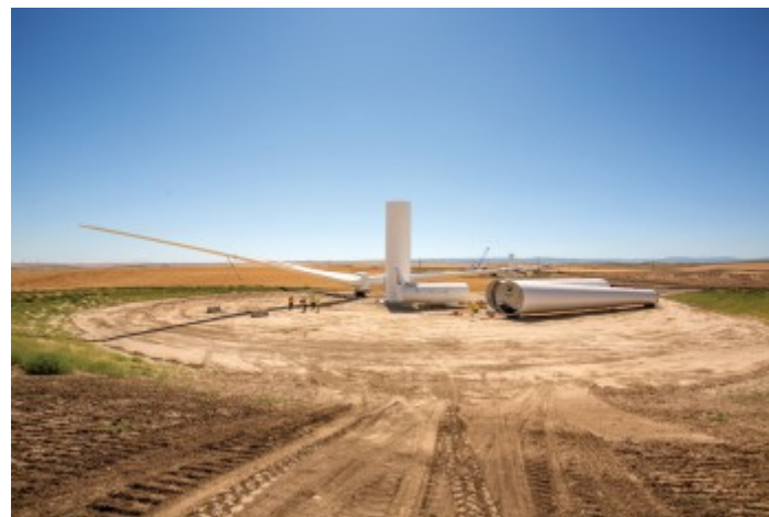
Tucannon wind farm, under construction Photos from: RES Americas
