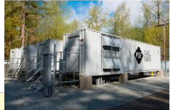
2 MW / 4.4 MWh lithium- ion/phosphate battery – Glacier, WA
