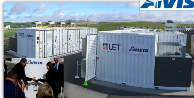
1 MW / 3.2 MWh UET vanadium-flow battery – Pullman, WA
