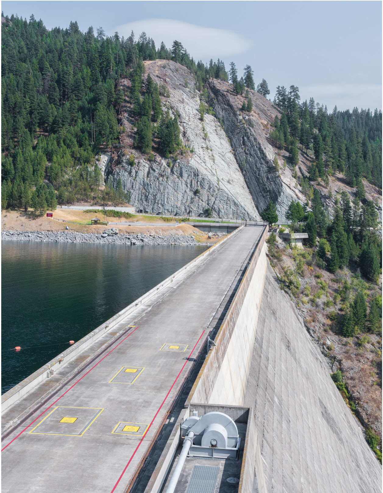
Libby Dam, photo by Tony Grover
