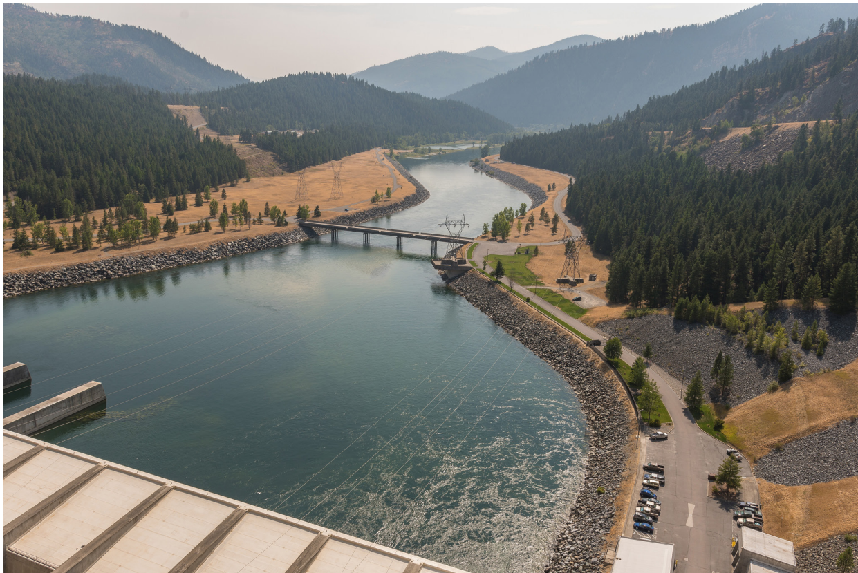
Libby Dam looking downstream at the Kootenai River, photo by Tony Grover
