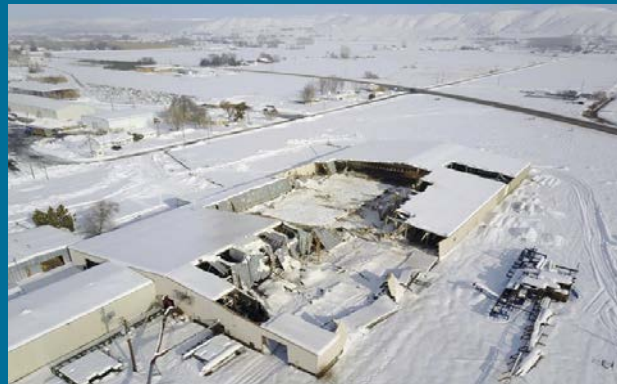
The Partners Produce facility in Payette, Idaho, collapsed under the weight of snow. (Jason Brainerd/Rapid Aerial LLC via AP)
