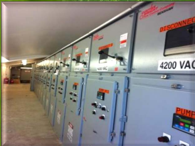
Electrical Panels, Variable Frequency Drive
