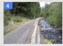
4 Example Ecological Concern: Streambed Channelization
