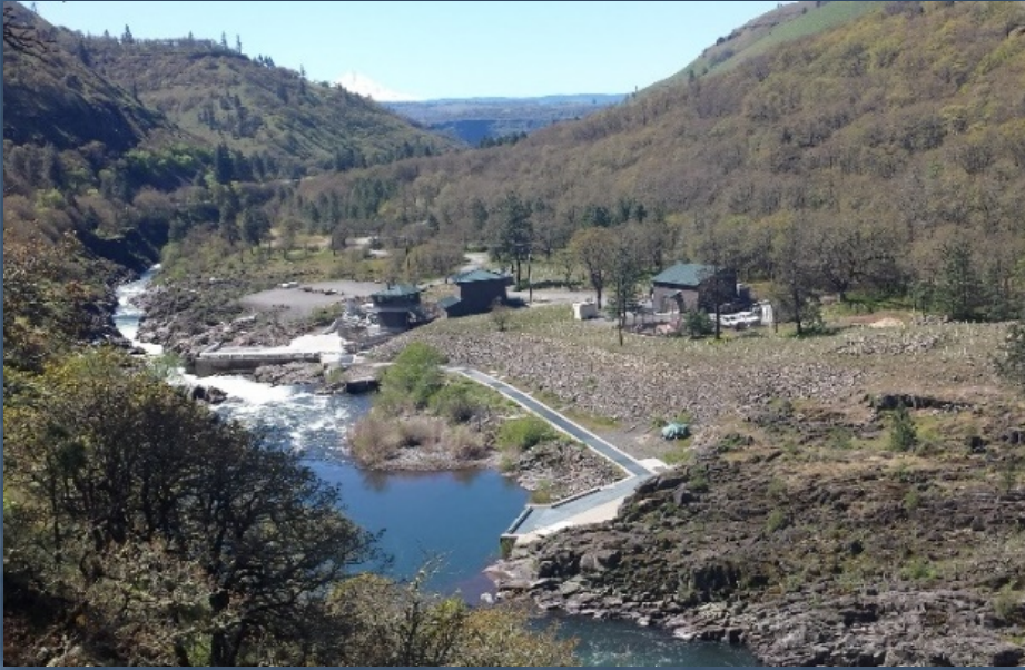
Lyle Falls Monitoring & Collection Facility
