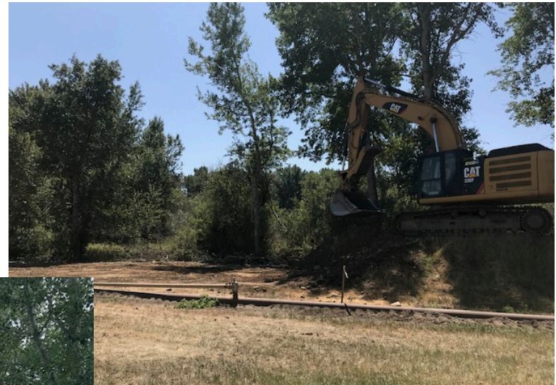
Installing the core of the berm
