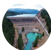
Tieton Hydroelectric Project (15 MWe)
