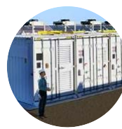
Horn Rapids Solar, Storage & Training Center (4 MWe)
