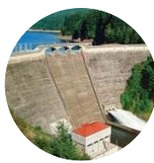
Portland Hydroelectric Project (37.5 MWe)
