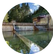
Packwood Lake Hydroelectric Project (27 MWe)
