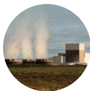
Columbia Generating Station (1,207 MWe)
