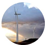
Nine Canyon Wind Project (96 MWe)
