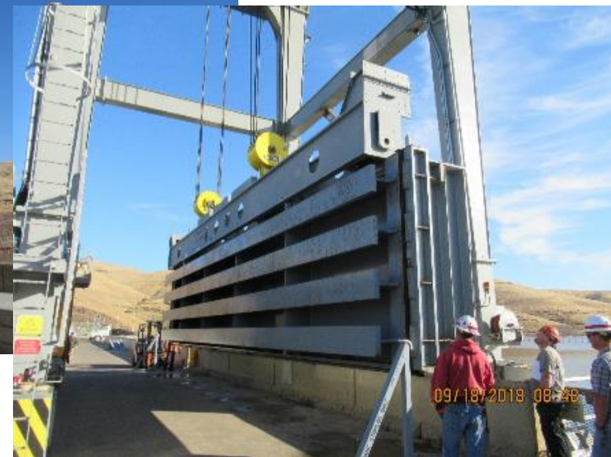
Stop Log Section
