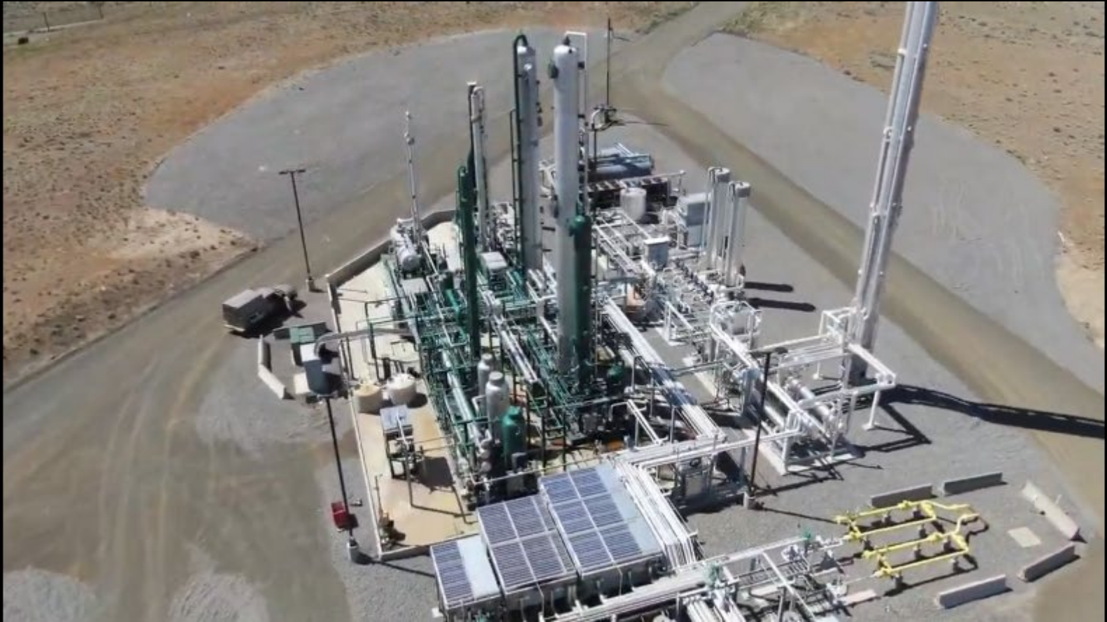
Aerial view of H.W. Hill Renewable Natural Gas Plant
