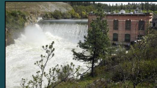
Nine Mile Dam, Avista Corp
