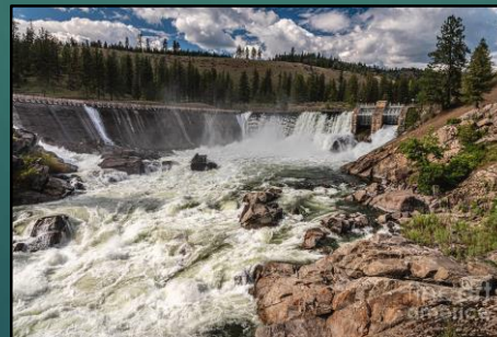
Little Falls Dam, Avista Corp.
