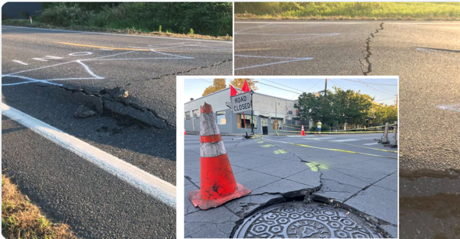
The intense Portland heat has caused streets and sidewalks to buckle. (AccuWeather/Bill Wadel)
