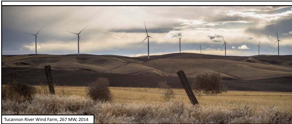
Tucannon River Wind Farm, 267 MW, 2014
