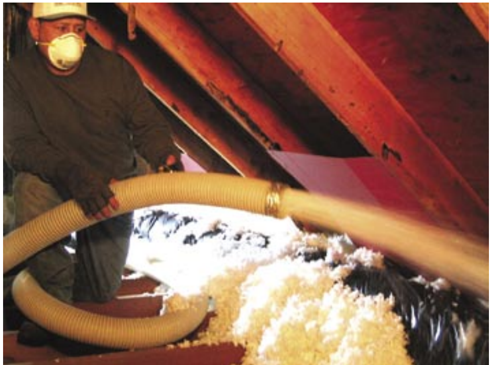
Crew member from Home Visions West blows insulation into an attic.
