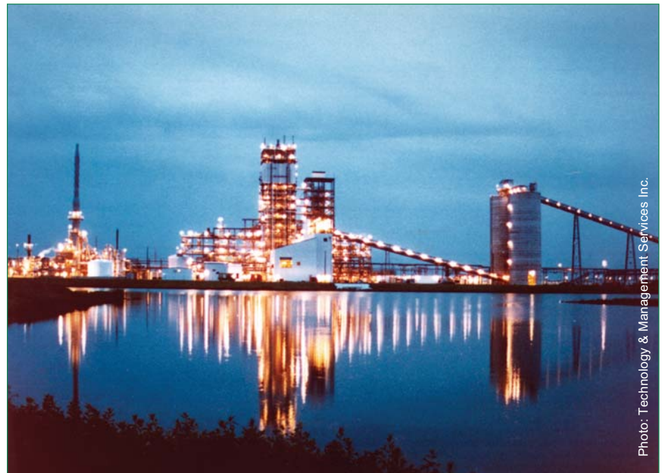
Tampa Electric's Polk Power Station, an integrated coal gasification, combined-cycle (IGCC) power plant.
