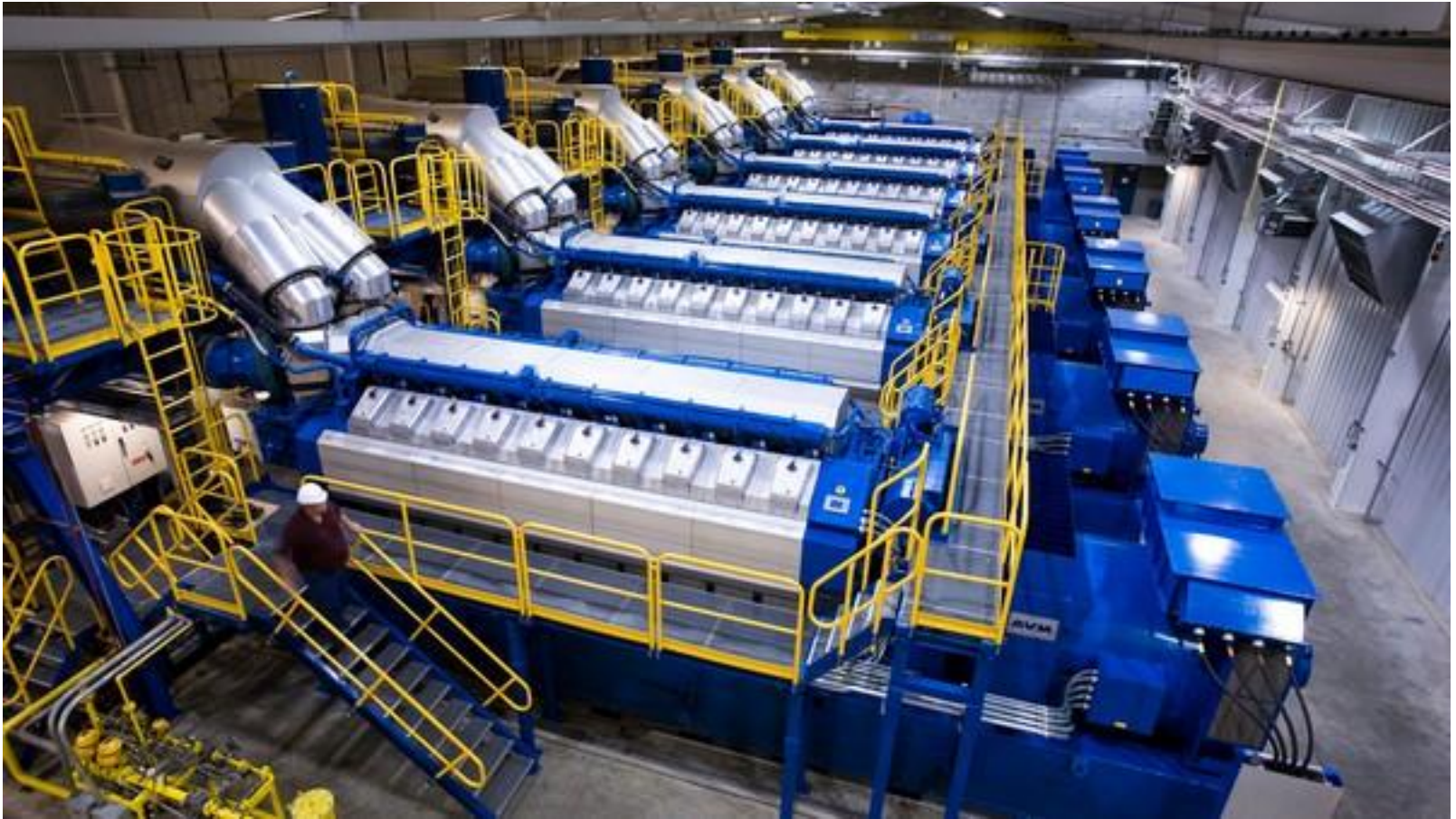
Engine Hall at Goodman Energy Center Kansas
